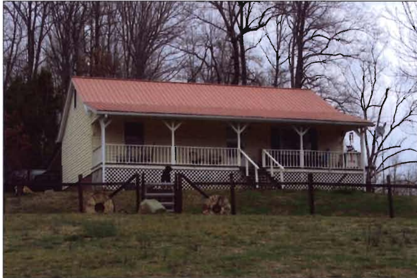
Property #2: House, 3464 Dickey Mill Road, PIN 9807814758
