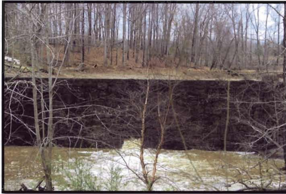
Dickey Mill, dry-laid stone dam, Penne Sandbeck (March 2009)
