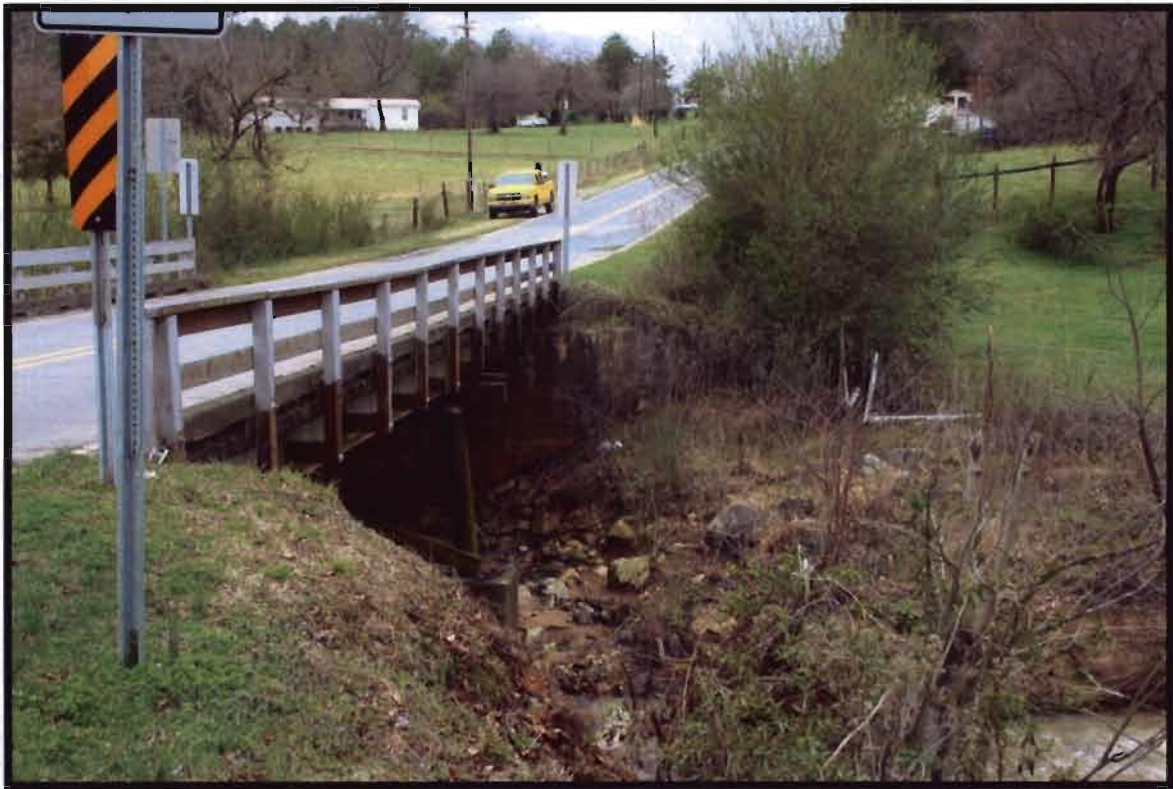
Bridge No. 64, North Elevation, SR 1912 over Quaker Creek, Penne Sandbeck, (March 2009)
