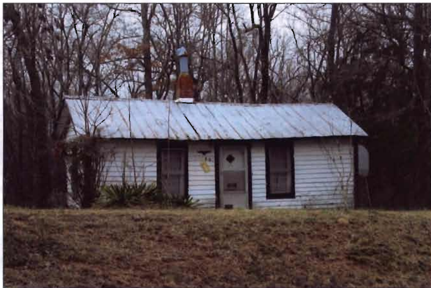
Property #3: House, 3601 Dickey Mill Road, PIN 9807915753
